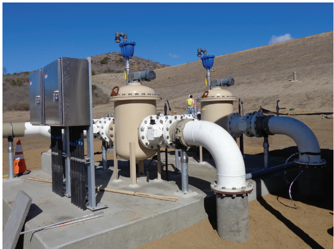
A view of the control panels on a 14" automatic strainer removing zebra mussels from lake water
